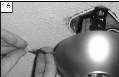
16 Make wire connections to power source using wire nuts provided. Make sure that no filaments are outside of the wirenut. After making the wire connections, the wires should be spread apart with the grounded conductor and the equipment-grounding conductor on one side of the outlet box and ungrounded conductor on the other side of the outlet box.
